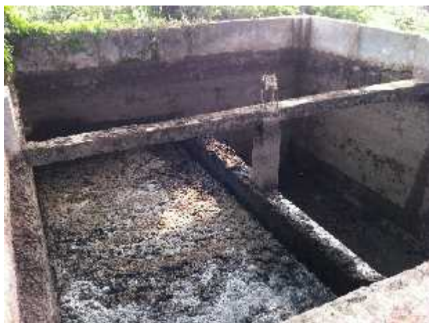
Picture 2-2: Poultry feces collection and storage chamber
